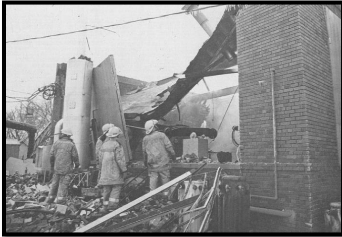
RVFD surveying the damage after the 1989 Light Plant explosion
