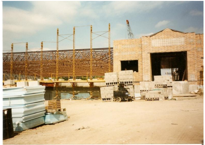
Construction on the new Randolph High School
